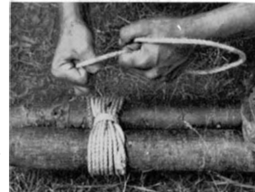
Make two complete frapping turns around lashing turns between the timbers.
