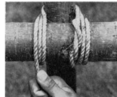
In wrapping, the rope goes on outside of previous turn around crosspiece, on the inside of previous turn around upright.
