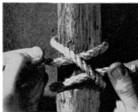
Pass rope end around the pole again below the first turn. Bring the end under the rope.
