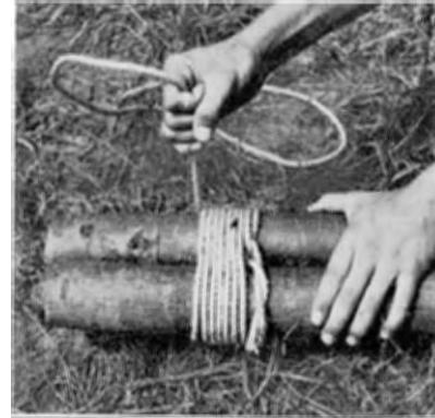
Bind timbers together by seven or eight turns. Make turns loose, one beside the other.
