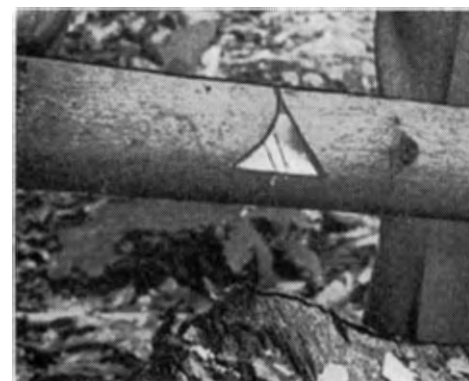
The cleaned-out notch is ready for a fitting—round stick or dovetail.
