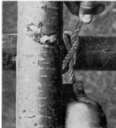
SQUARE LASHING: Start with a clove hitch around upright, just under the spot where crosspiece is to be.
